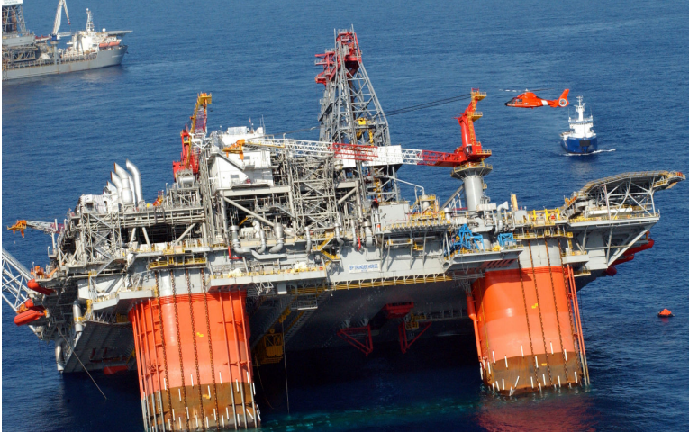
Figure 1.1: A semi-submersible oil platform, Thunder Horse, was found listing after hurricane Dennis had passed through the region in 2005. Photographed by U.S. Coast Guard.
